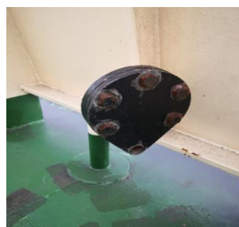
Hydrant connection type DN50, PN16.
